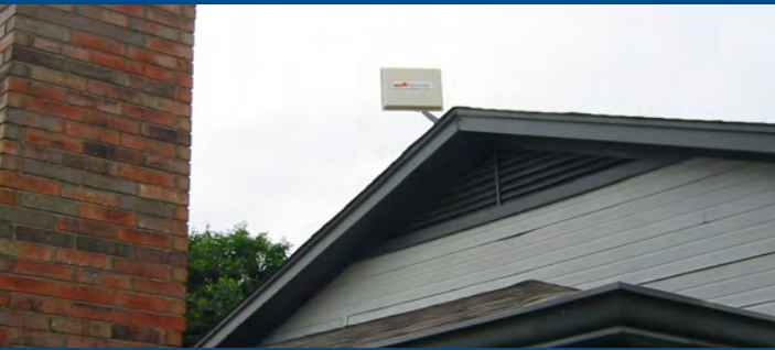
This small home-based antenna is typical for fixed wireless-access reception at low microwave frequencies. System installations at 28GHz are even smaller. (Source: Wikimedia Commons)
